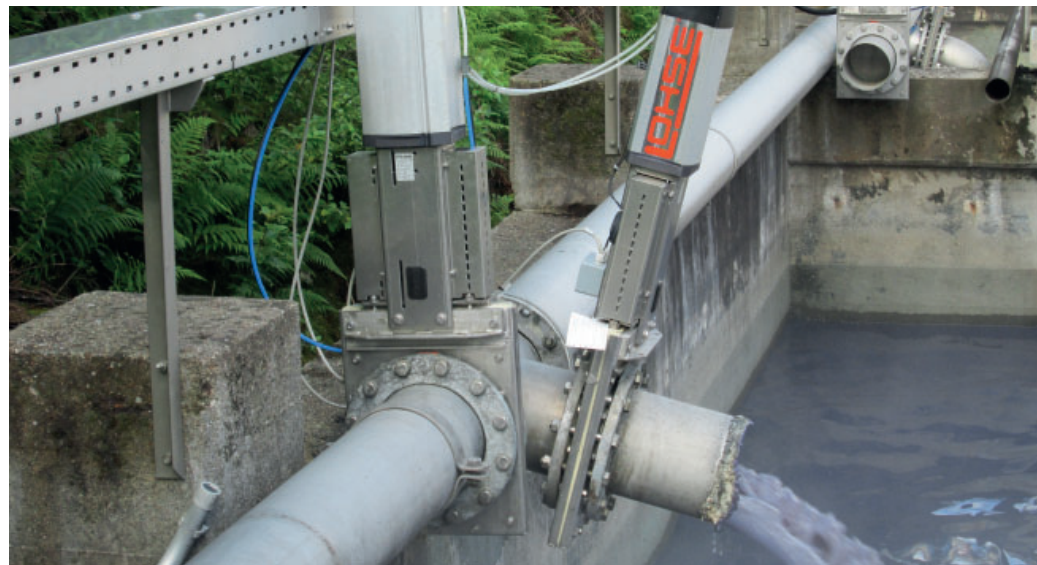
MARTIN LOHSE developed the CAW type gate valve especially for use in wastewater treatment. Non-corrosive materials make it possible to withstand the adverse conditions.
