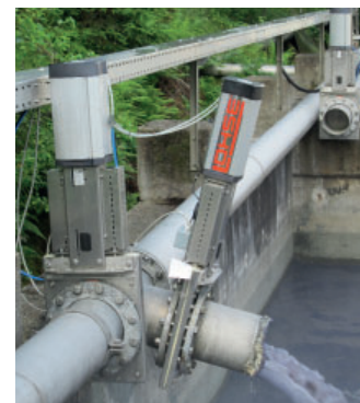
Gate valves from LOHSE control the flow of waste water, for example.
