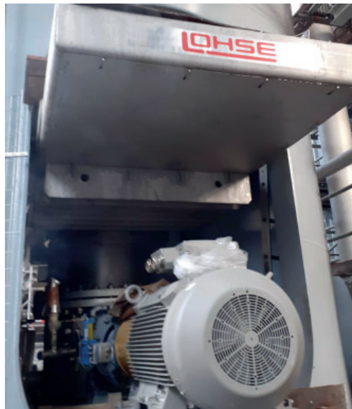
DN1200 outlet valve with electric actuator under a 35 m high pulp tower.
